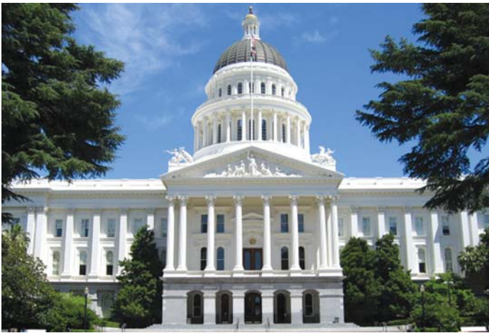
At the State Capitol, we advocate for the Pipe Trades.
